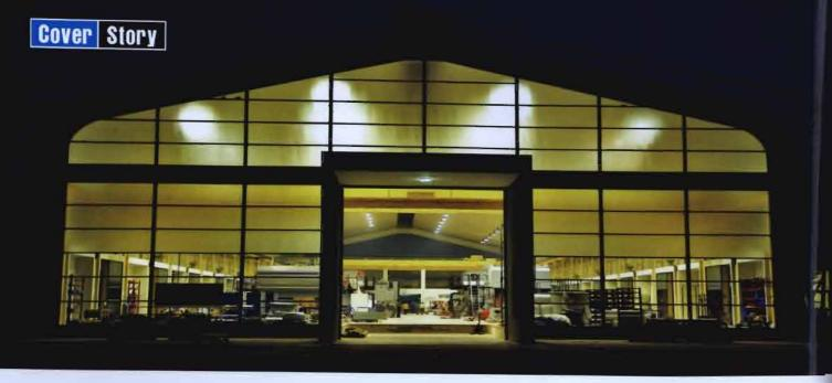
addition to meeting the functional challenges, the use of steel as the construction material helped to meet the time constraints of the project. While the steel super structures were prefabricated, the concreting work for the foundation was carried out simultaneously. The modularity of design, choice of material and efficient project management helped complete the project within a short time frame.
