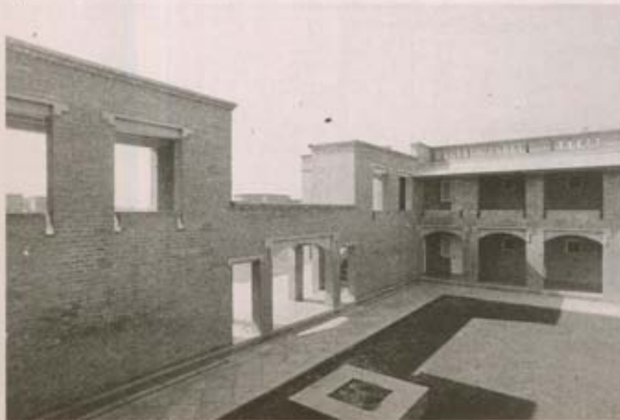
Open-to-sky courtyard in the hostel block
