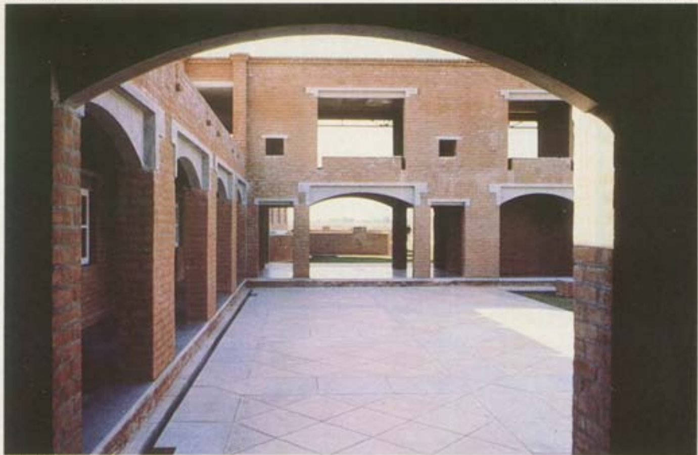
Open-to-sky paved court
