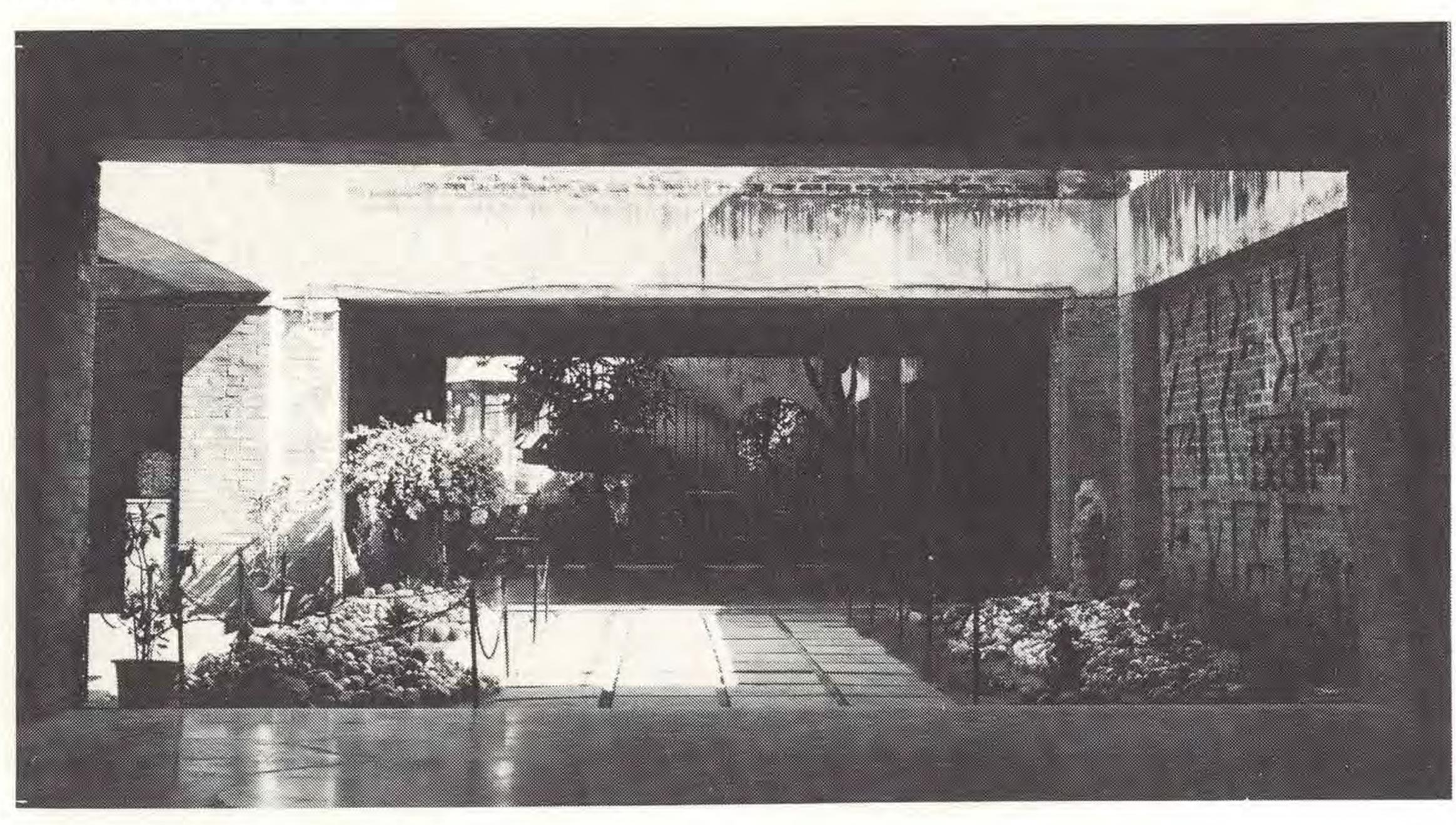
rooms and circulation areas, thus encouraging activities to spill out onto corridors and courtyards. The structural system consists of cruciform brick columns tied at the top by channel beams of reinforced concrete. Larger spaces, such as the multi-purpose hall, are composed of four grid units, with the central column omitted and a roof of four funicular shells supported on internal cross-beams. Murals, created of brick and concrete, form the visual focus of courtyard spaces.
